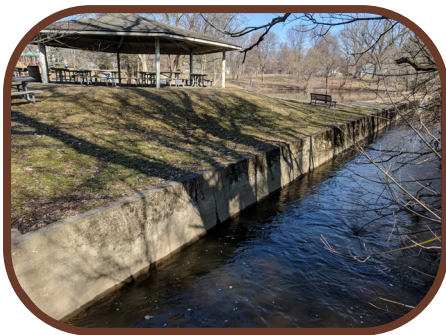
Concrete wall channelizing creek
